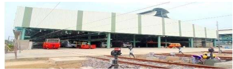
Construction of Metro Rail Depot, Kalindi Kunj, New Delhi
