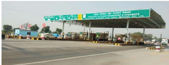
Development & Operation of Bikaner-Suratgarh Section of NH-62 (earlier NH-15) in the state of Rajasthan
