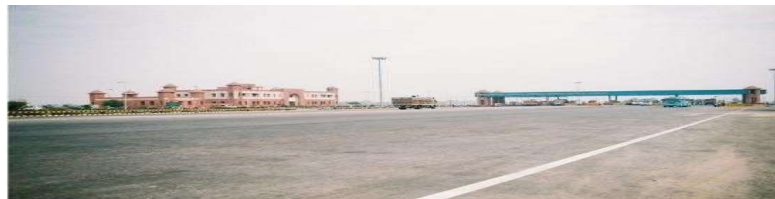
Toll Plaza construction at Delhi –Agra, NH-44 (earlier NH-2)
