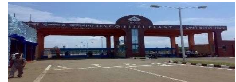
Approach Road 2 lane from GT Road at Neamatpur to Burnpur, West Bengal
