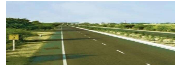
4 laning at Agra- Gwalior section, NH-2, in the State of Madhya Pradesh
