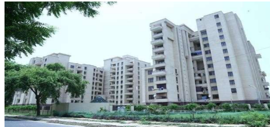
Residential accommodation for NHA staff at Sector 17, Dwarka, New Delhi
