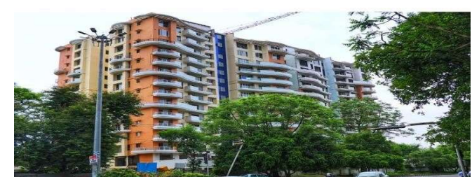
Construction of 96 flats at Tulsi Tower, Bhopal for MP Housing & Infrastructure Development Board
