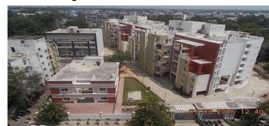
Construction of 92 flats at Mahadev Towers, Bhopal for MP Housing & Infrastructure Development Board
