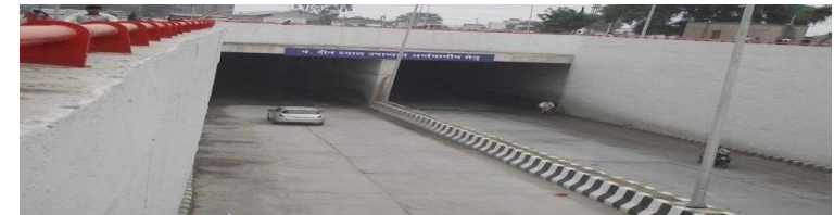
Construction of RUB at Badli, New Delhi
