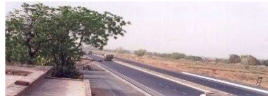
4 lane of km 41-51 of Agra Dholpur of NH-46 (earlier NH 3), in the state of Rajasthan
