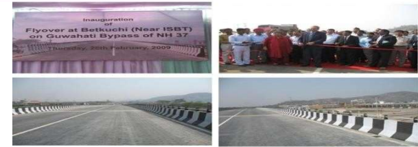
Construction of 2 lane flyover on Guwahati Bypass of NH-115 (earlier NH-37) in the state of Assam
