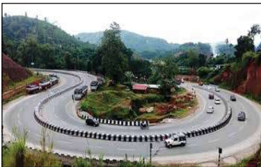
Roads & Highways Construction /EPC
