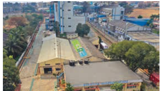
Bengaluru Plant Manufacturing facility for Adhesives & PU Resins
