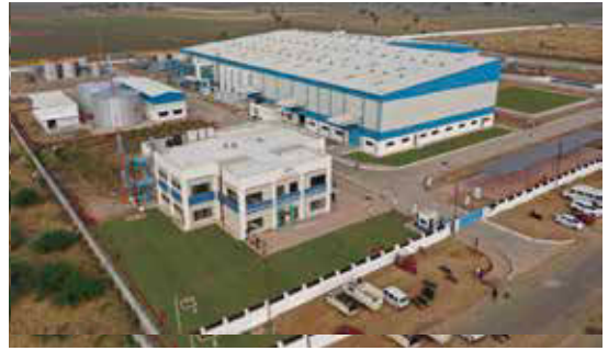
Saykha Plant Manufacturing facility for Liquid Inks
