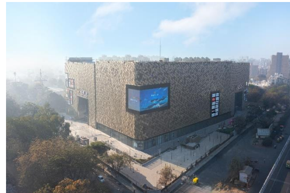
Palladium Ahmedabad Feb-23
