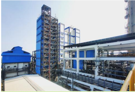
Nitric Acid plant
