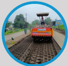
Compaction by Pad Foot Roller
