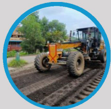
Grading & Profiling with motor Grader
