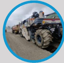
Pulverization of soil with Recycler
