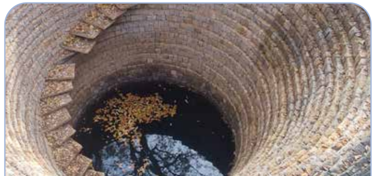
Open well harvests rainwater, & recharges groundwater. The Manu Vadar traditional well digger community was involved in creating this well. Lalbagh Botanical Garden, Bengaluru, Karnataka
