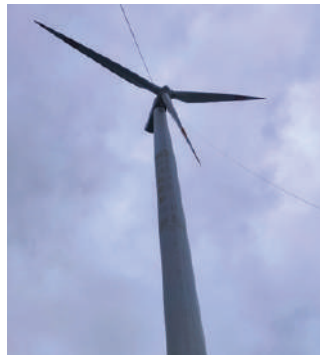
1.5 MW Wind turbine
