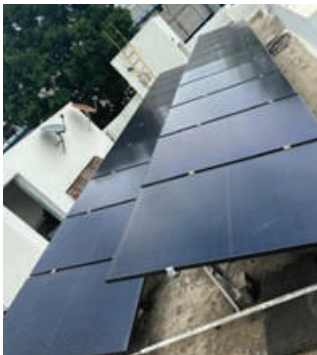
4KW solar rooftop installation
