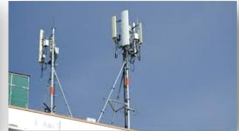
Roof Top Tower
