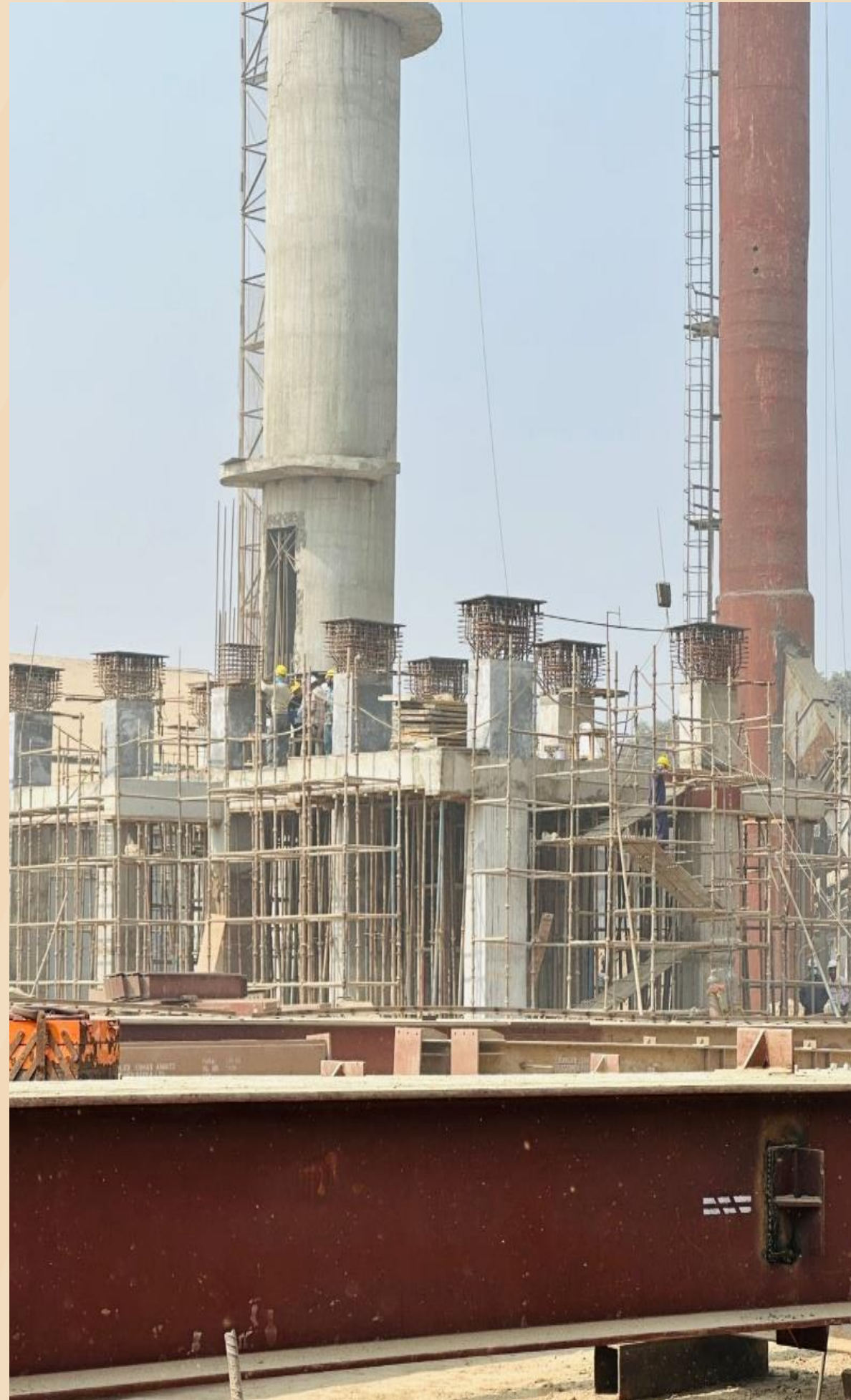
Recovery Boiler Upgrade
