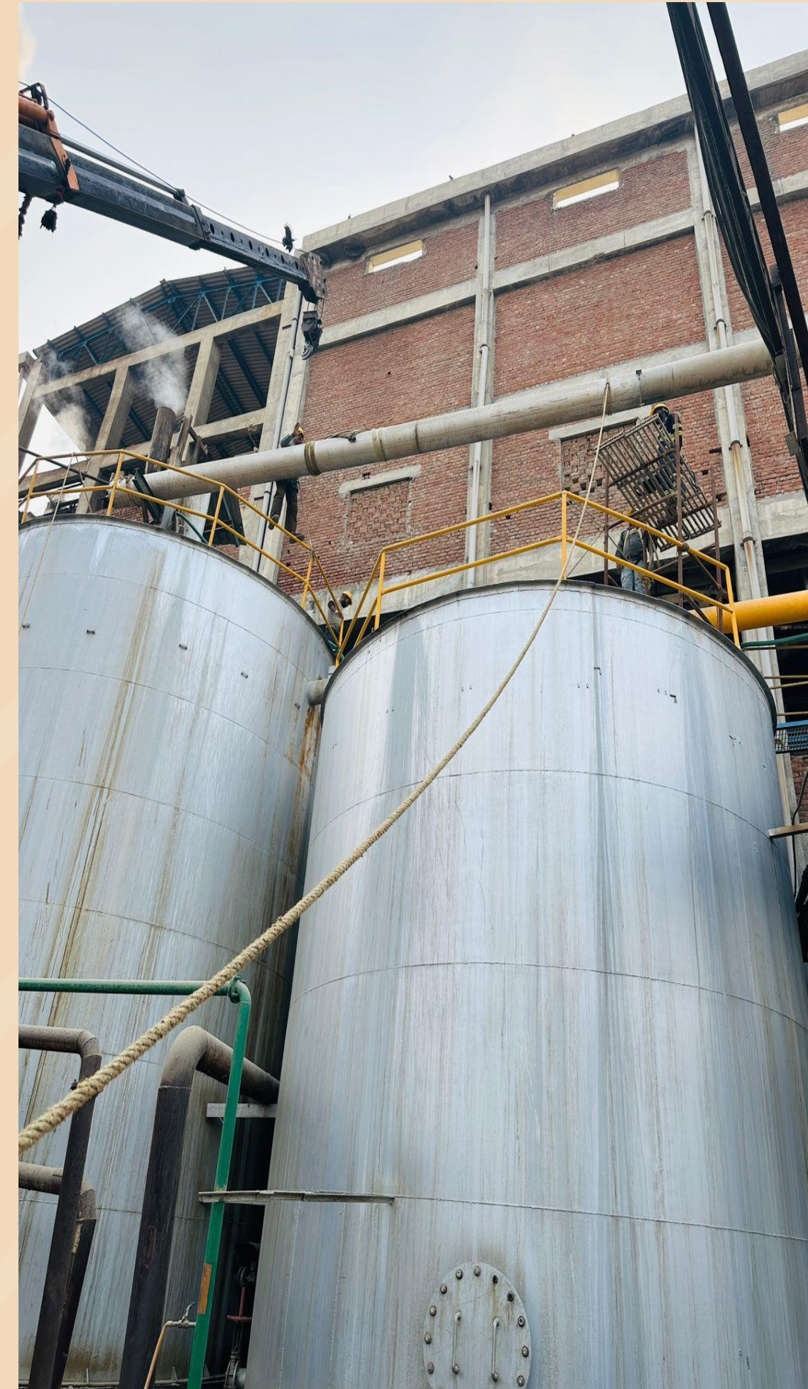
Pulp Mill Upgrade
