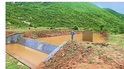
Water Conservation Project
