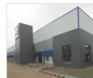
Foundry Division, Vambori
