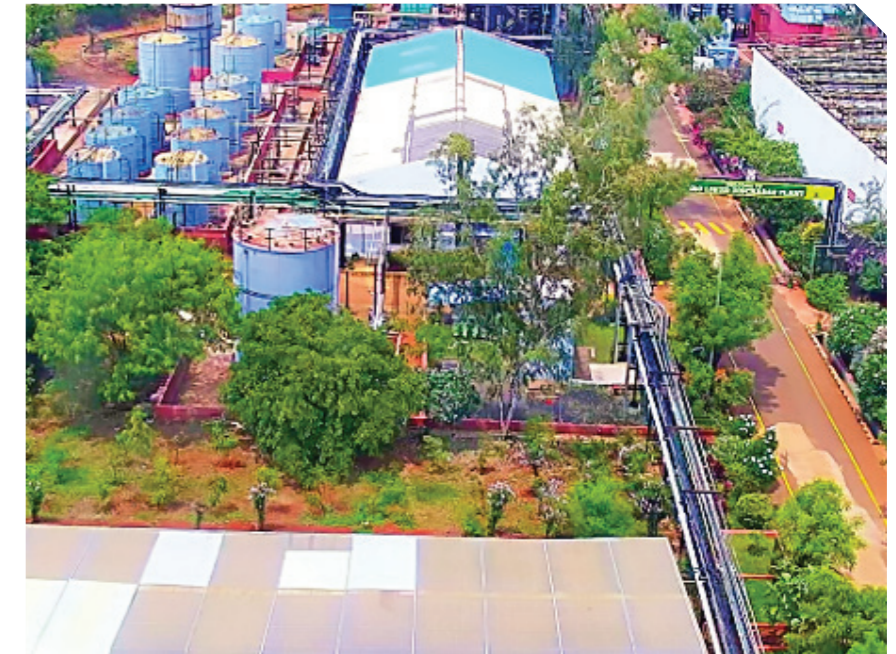
➤ Zero Liquid Discharge plant, Digwal, India
