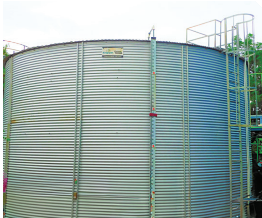
➤ Rainwater collection system, Digwal, India
