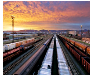
Dedicated Freight Corridor
