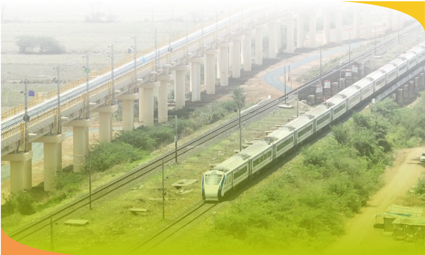
▲ First Rail over Rail (ROR) by RVNL-2.2 km long rail flyover near Gudur Railway yard, SC Railway
