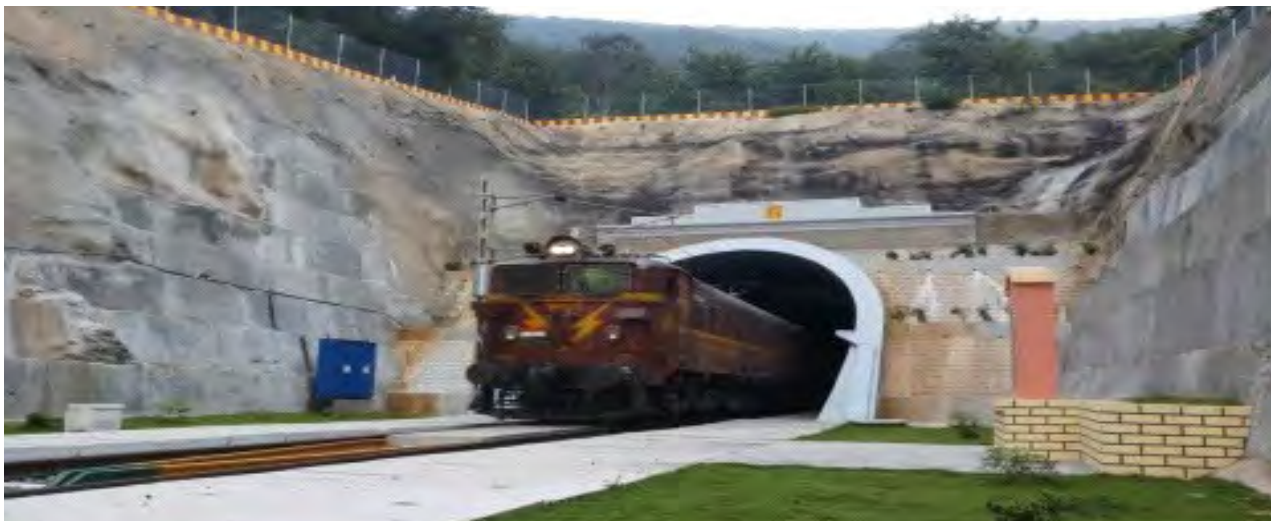
Tunnel on KRCL Line
