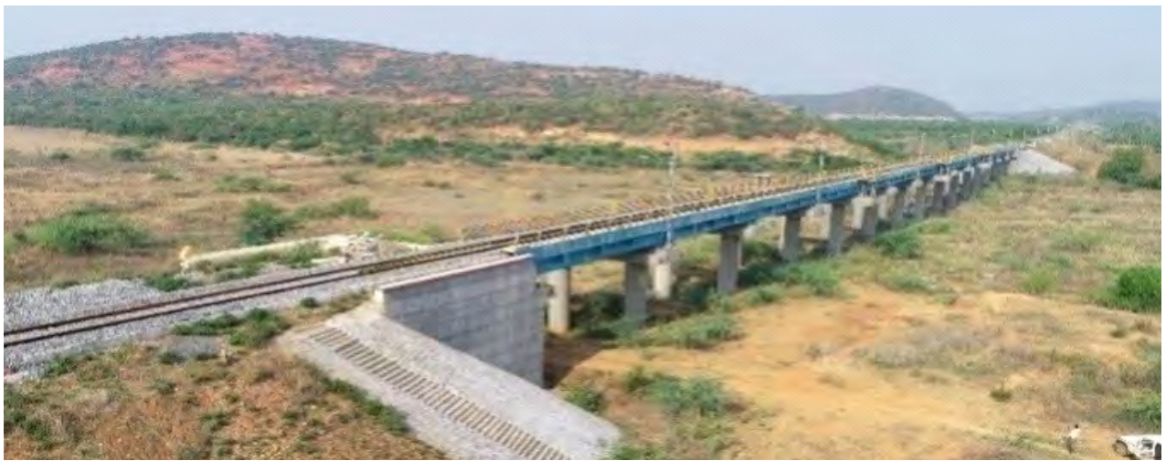
New Rail Line between Krishnapatnam & Obulavaripalle
