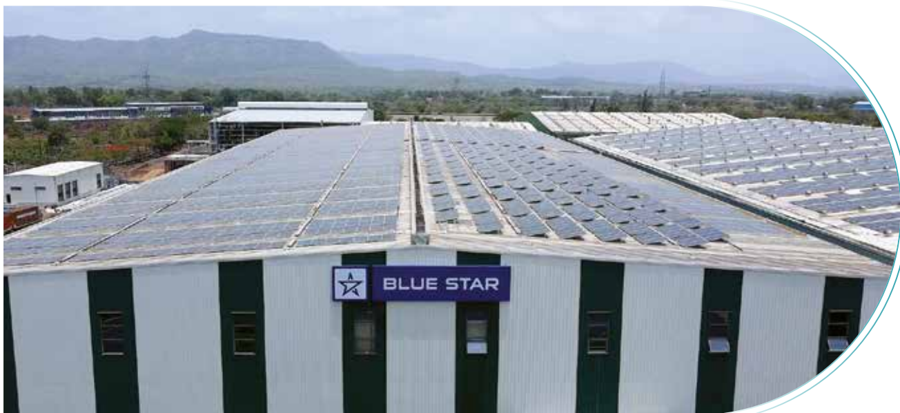
3.1 MW rooftop solar facility at Wada Plant
