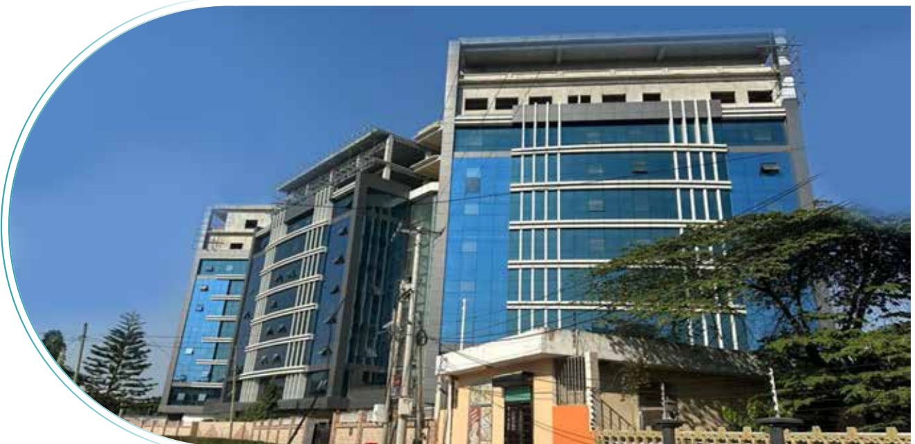
VRF system supplied at Shifa Hospital, Phase 2&3 in Tanzania
