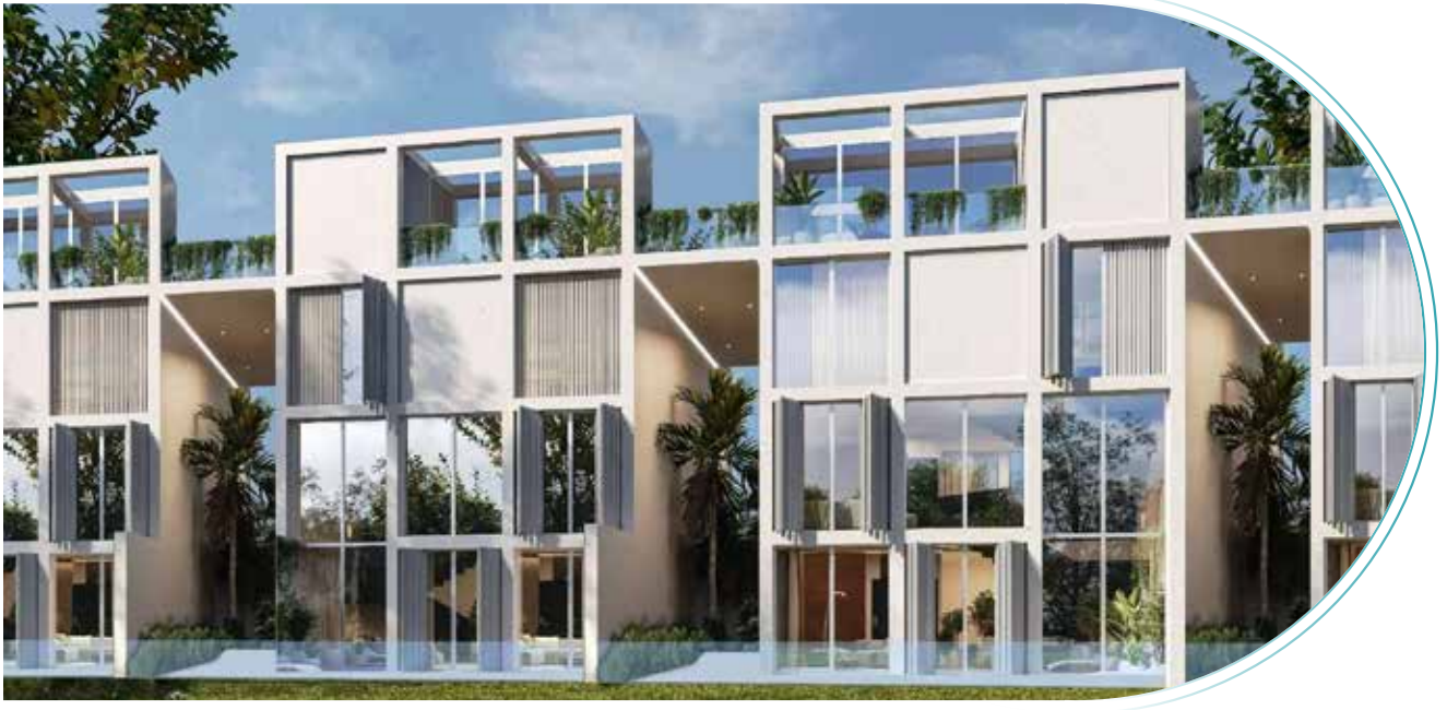
Supply of VRF system at Ixora Villas at Al Barari, UAE
