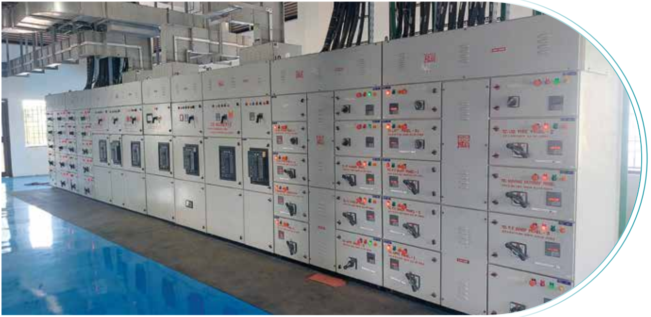
MEP works for Kilambakkam Bus Terminus, Chennai
