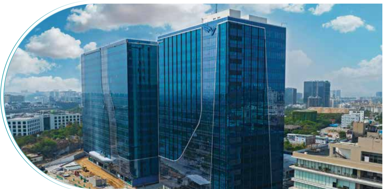
MEP works for Phoenix H10 Building in Hyderabad
