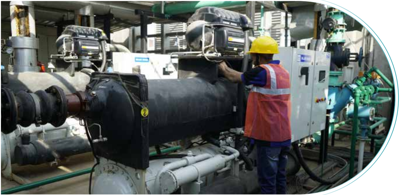
MEP works for Breach Candy Hospital, Mumbai
