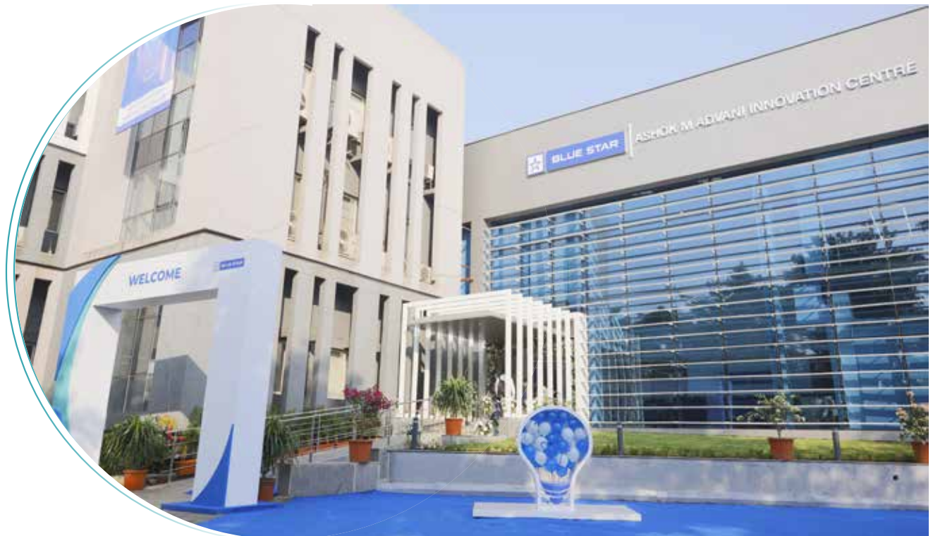
Blue Star's Ashok M Advani Innovation Centre located in Bhiwandi, Maharashtra
