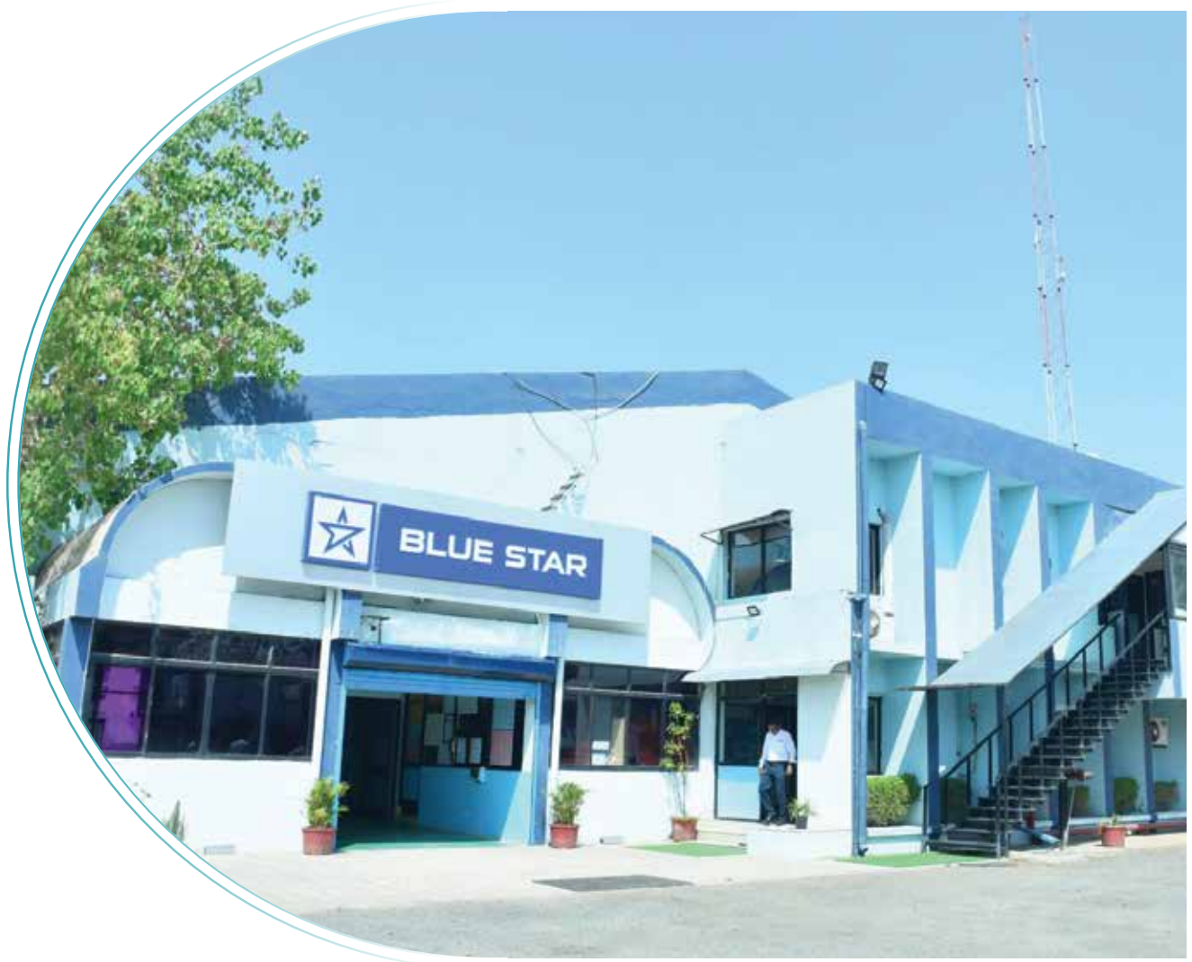
Blue Star's Ahmedabad Manufacturing Plant
