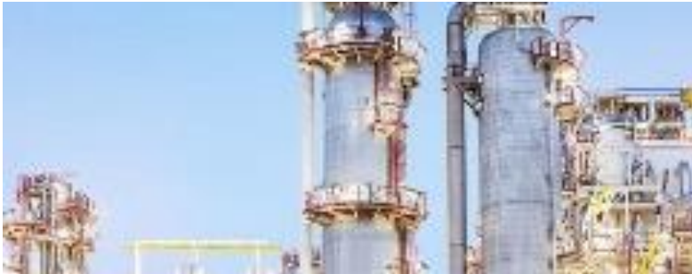
Smart control system for a major chemical manufacture in Hyderabad
