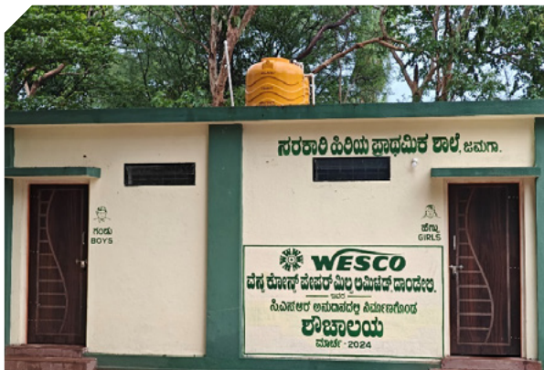
Toilet Blocks - Govt. Hr. Pr. School, Janga Village
