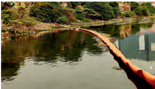
➤ Installed trash barriers, curtailing floating waste from falling into the Yamuna River, sustaining the local ecology
