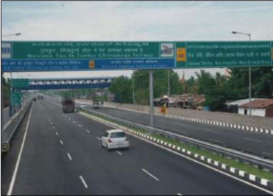
Figure 8-1 : General Condition of project road
