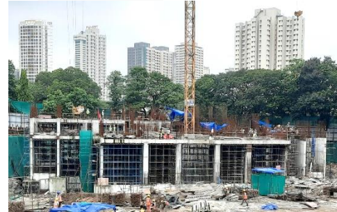
Tower (C) Ground floor slab work in progress
