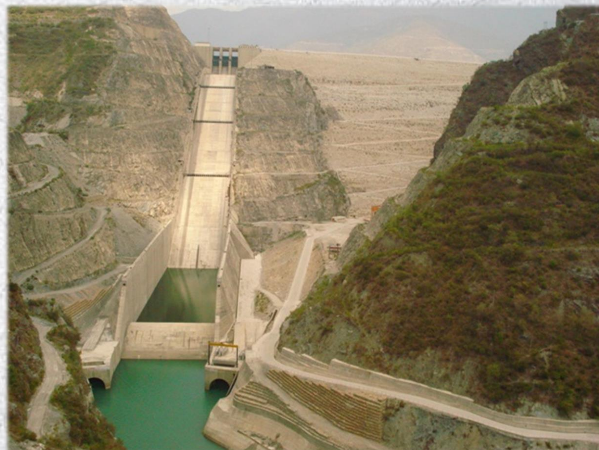
Tehri Dam, Garhwal
