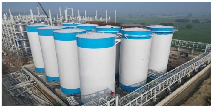
Tank Farm Area
