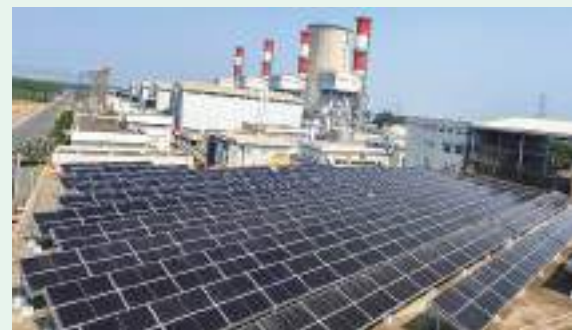
275 kWp Solar Rooftop at SUGEN Plant, Surat
