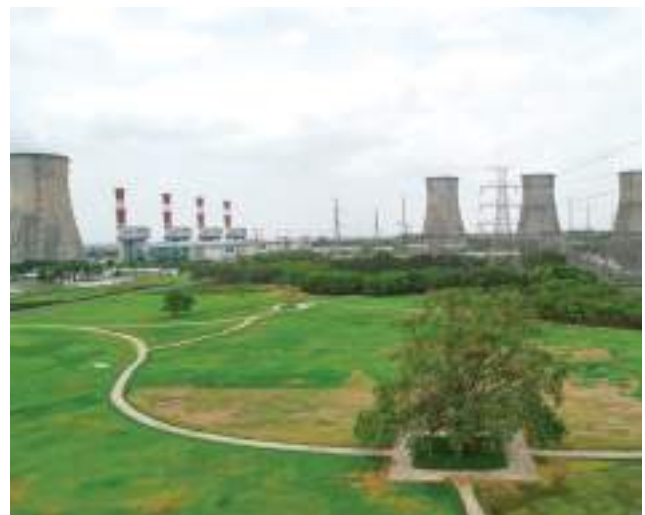
1,530 MW Gas-based SUGEN & UNOSUGEN Power Plants, Surat
