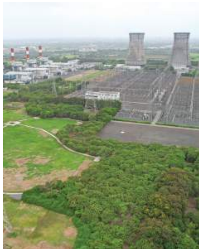
1,530 MW Gas Based SUGEN & UNOSUGEN Power Plants, Surat
