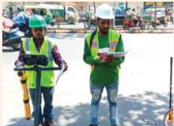
Underground Survey Using GPR at Ahmedabad
