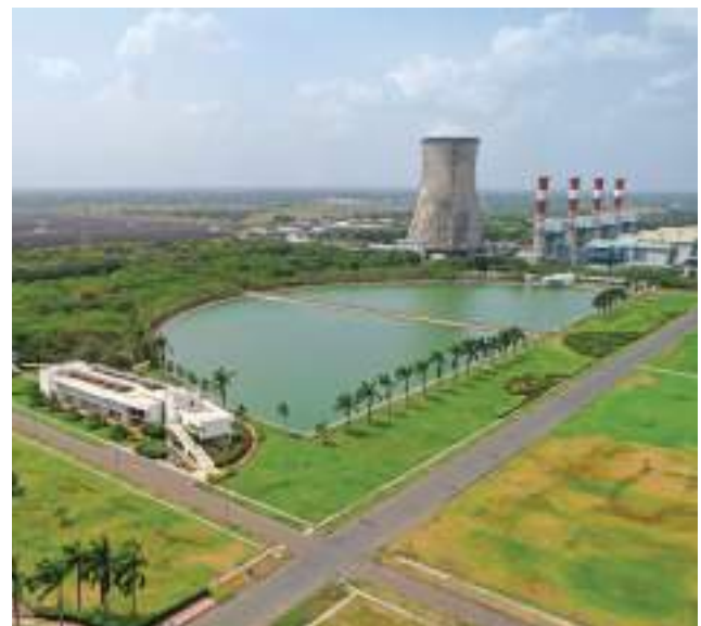
1,530 MW Gas Based SUGEN & UNOSUGEN Power Plants, Surat
