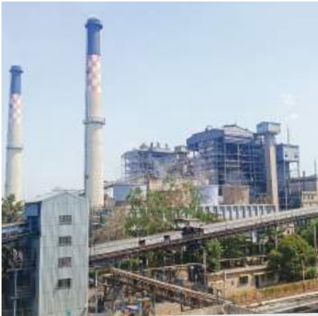
362 MW AMGEN Power Plant, Ahmedabad
