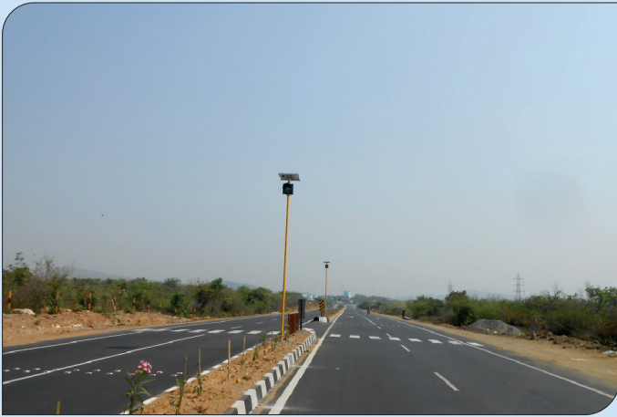
HKR Roadways Limited
