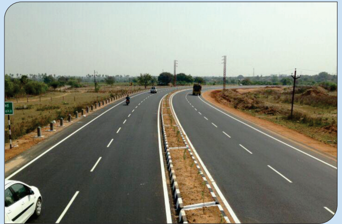
HKR Roadways Limited
