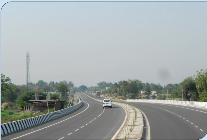
HKR Roadways Limited
