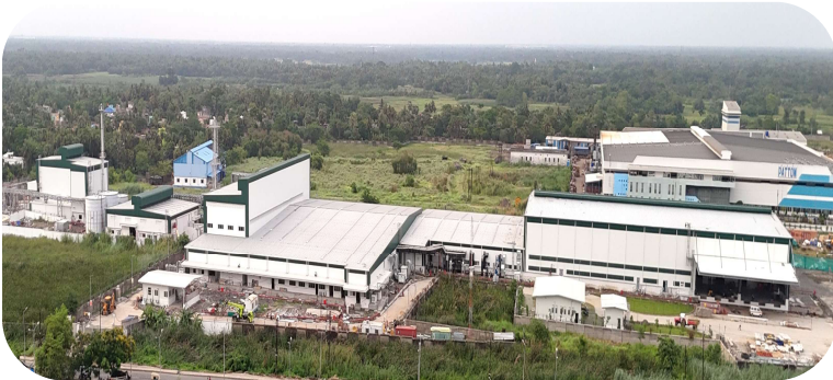
Personal Care Facility, Uluberia
