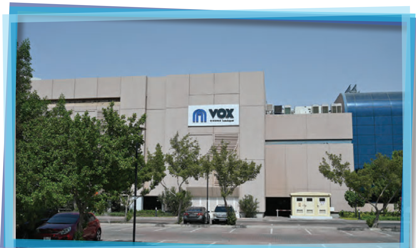
The Vox Cinema in Dubai, where Blue Star executed HVAC refurbishment and upgradation works
