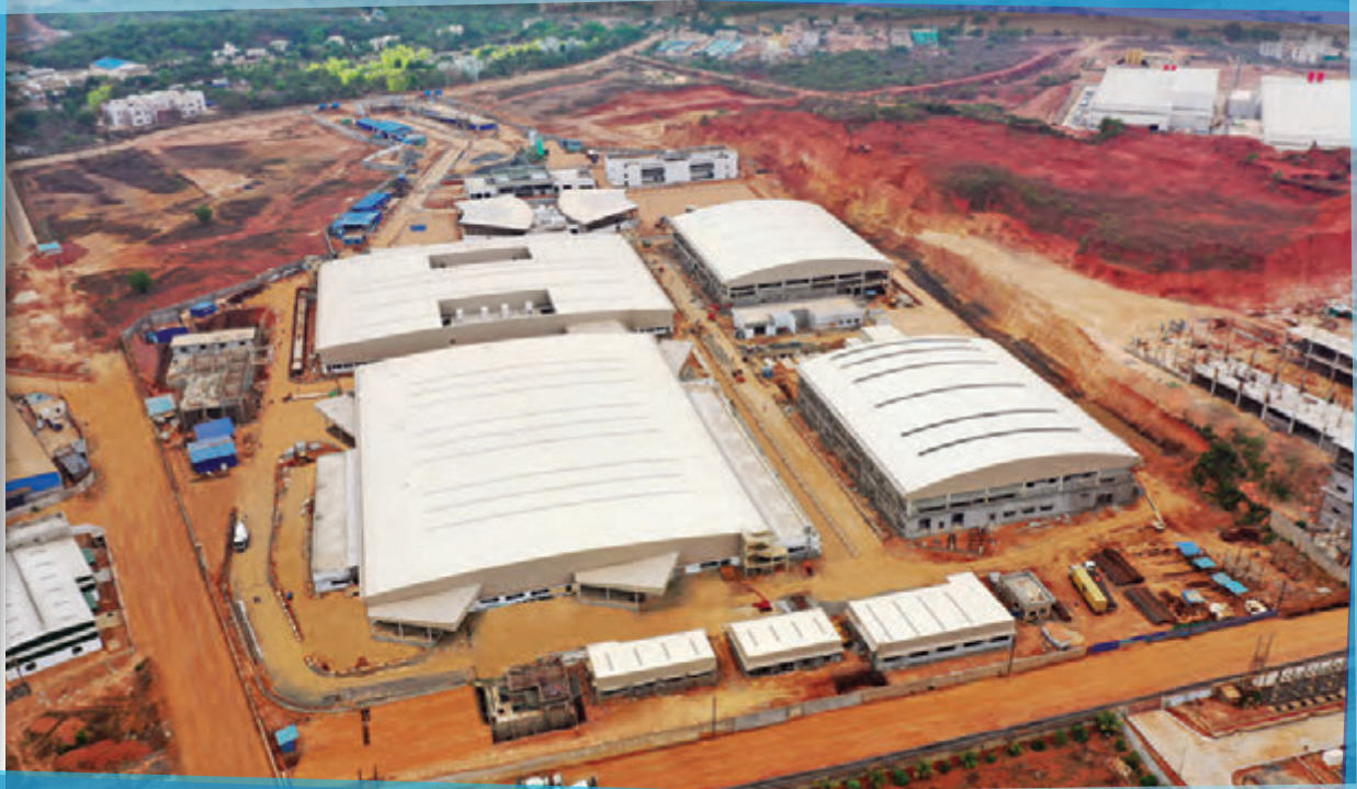
The Jockey factory at Cuttack, where Blue Star executed the HVAC, Fire-fighting and Electrical works
