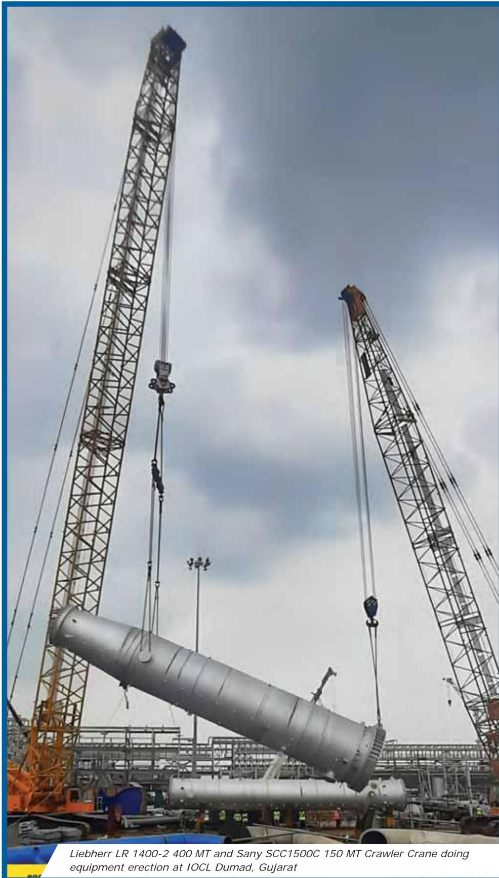
*Liebherr LR 1400-2 400 MT and Sany SCC1500C 150 MT Crawler Crane doing equipment erection at IOCL Dumad, Gujarat*
