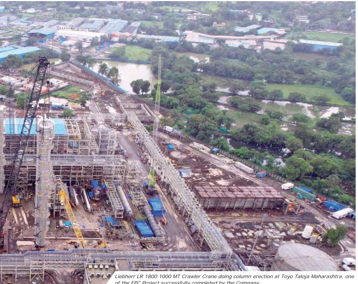
*Liebherr LR 1800 1000 MT Crawler Crane doing column erection at Toyo Taloja Maharashtra, one of the EPC Project successfully completed by the Company*
