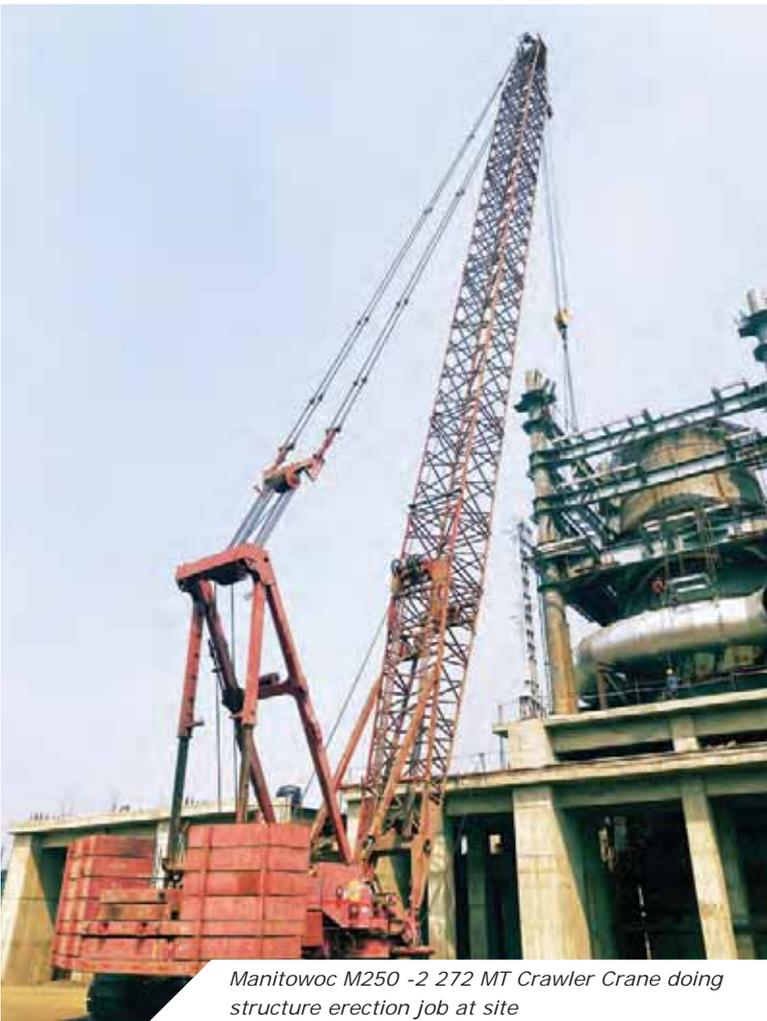
*Manitowoc M250 -2 272 MT Crawler Crane doing structure erection job at site*
