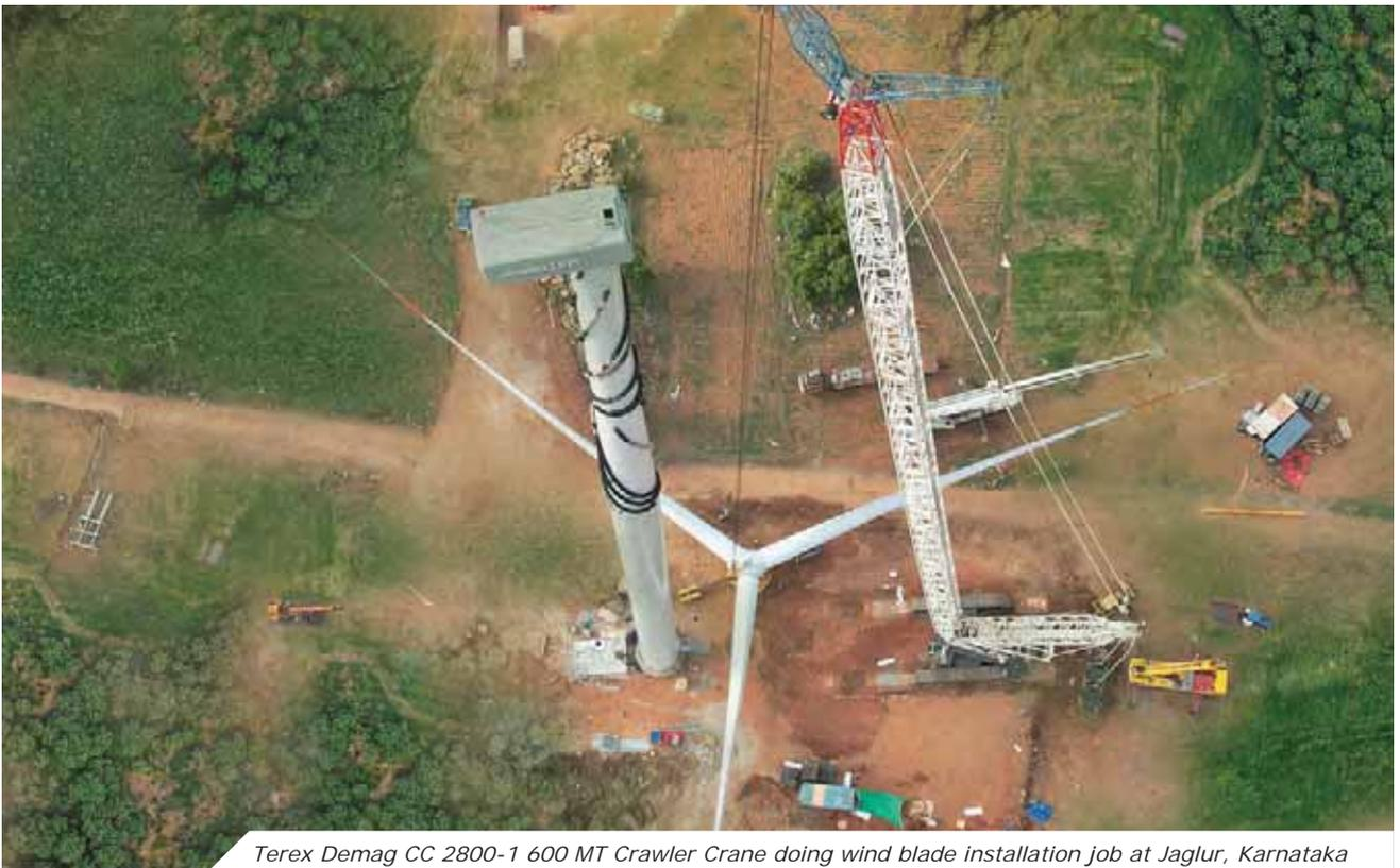
*Terex Demag CC 2800-1 600 MT Crawler Crane doing wind blade installation job at Jaglur, Karnataka*
