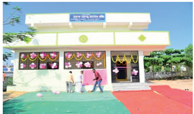
Construction of Mahila Bhavan.
