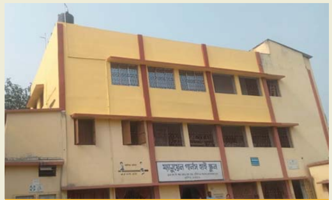
Creating infrastructure for auditorium Hall and facilities at Manuel Girls' High School at Budge Budge
