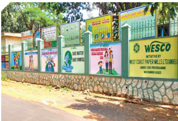
Compound Wall at Govt. Hospital - Dandeli
