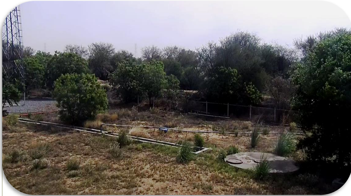
Rainwater harvesting system
