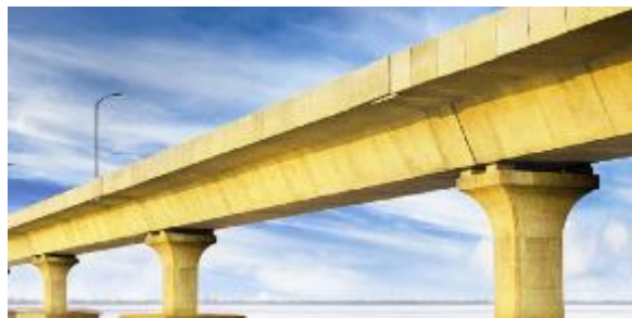
Dhola-Sadiya Bridge, Assam
