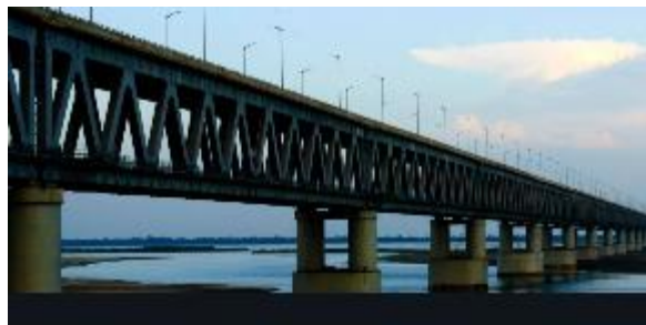
Bogibeel Bridge, Assam
