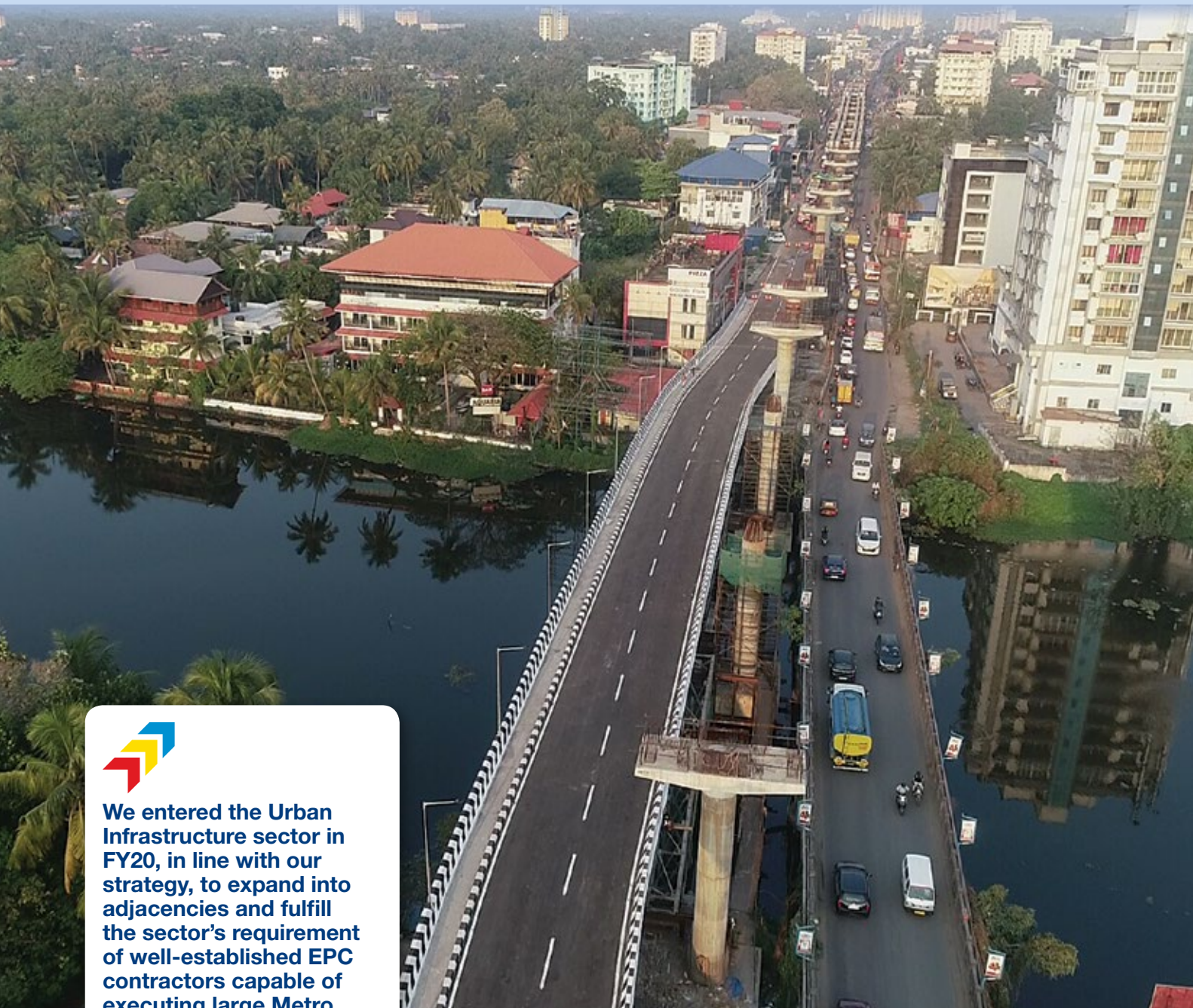
Kochi Metro and Panamkuttu River Over Bridge
