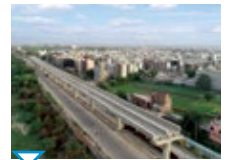
Delhi Metro Rail project, New Delhi
