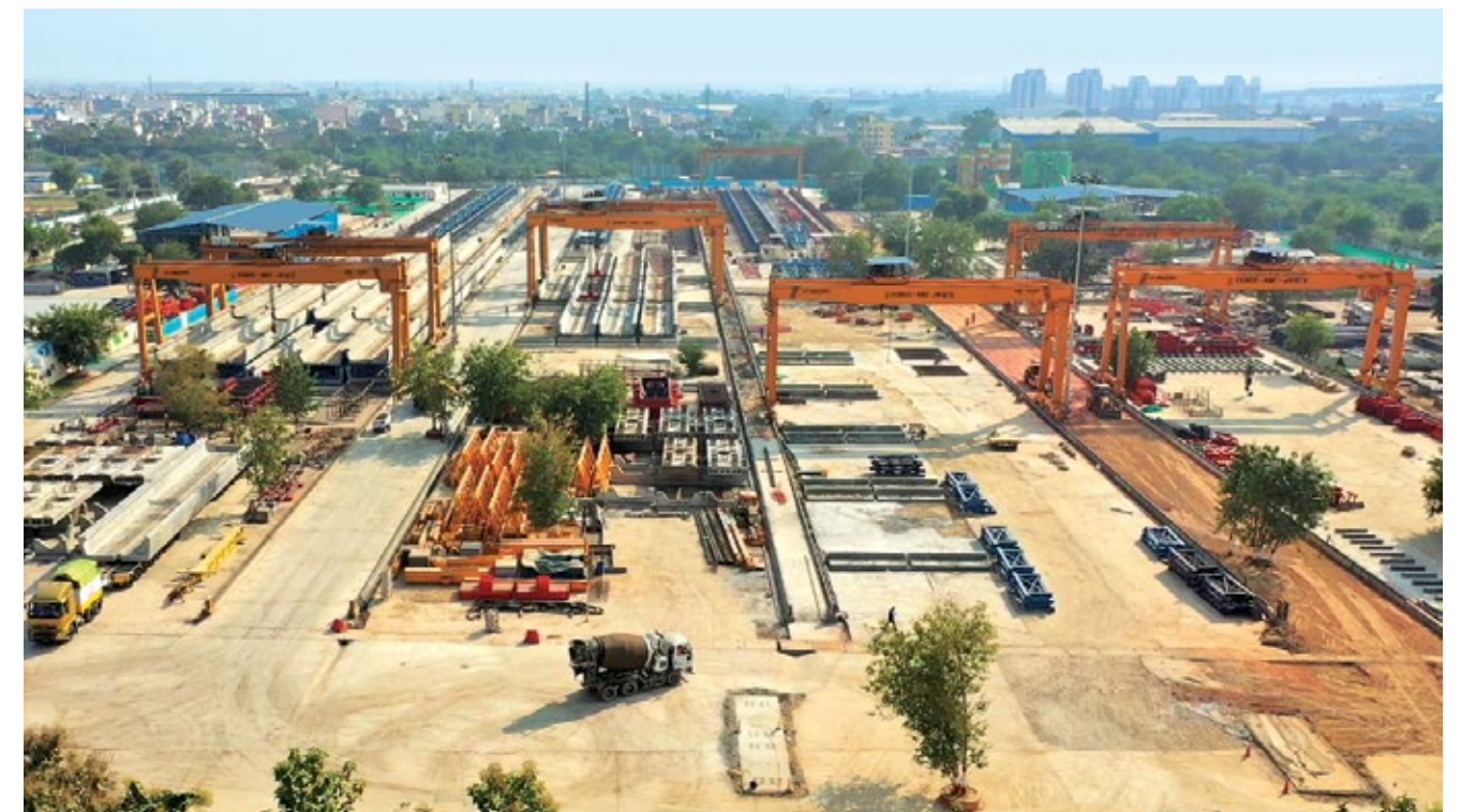
Casting Yard, Delhi Metro Rail project
