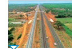
Third line between Gudur-Bitragunta, Andhra Pradesh
