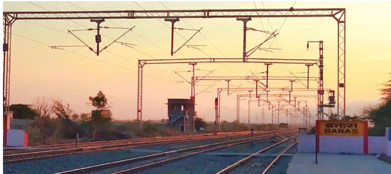
Rani-Swaroopganj Railway Electrification Project, Rajasthan
