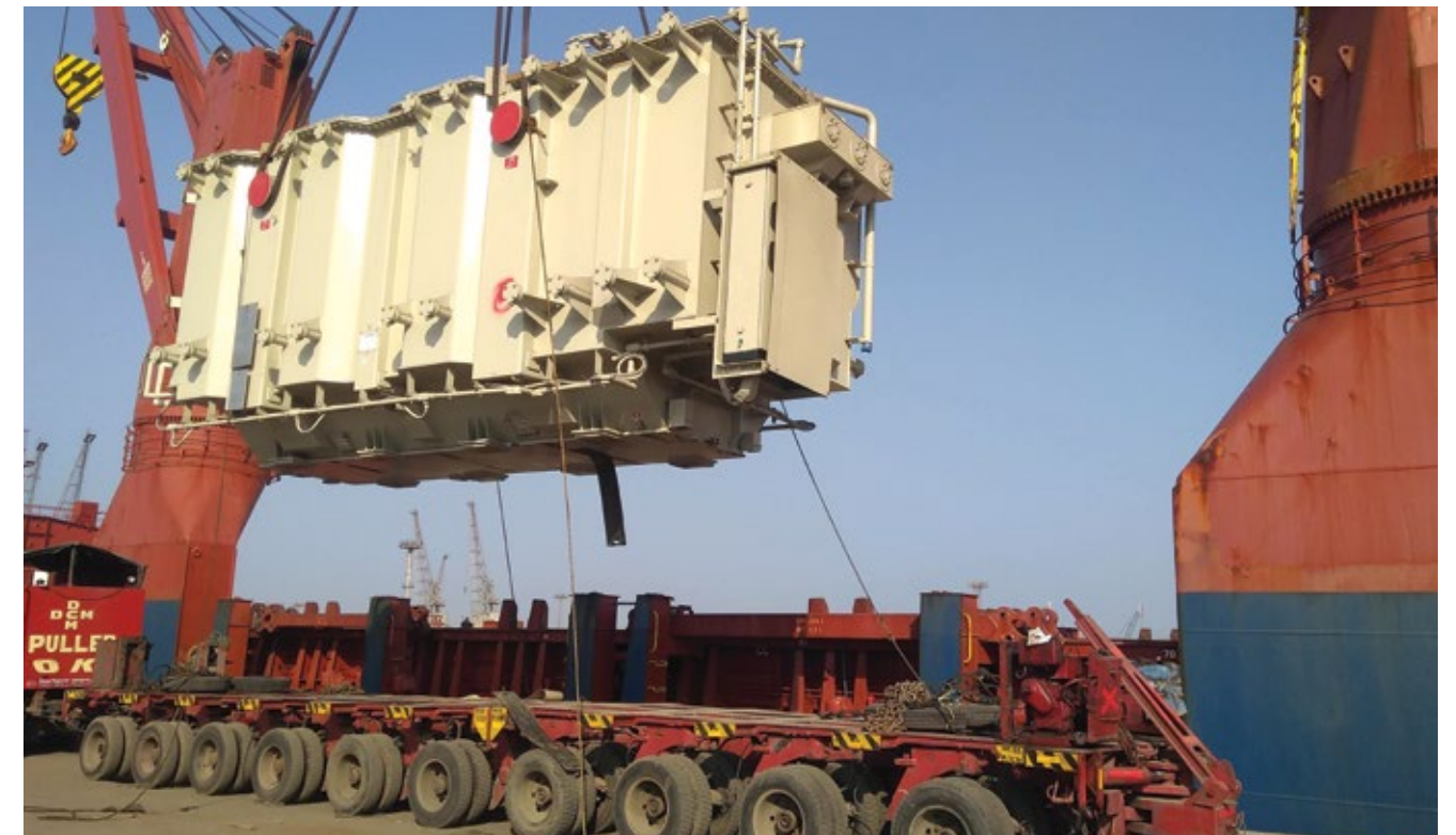
Despatch of material to project sites
