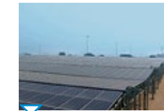
20 MW Solar Carport project, Haryana
