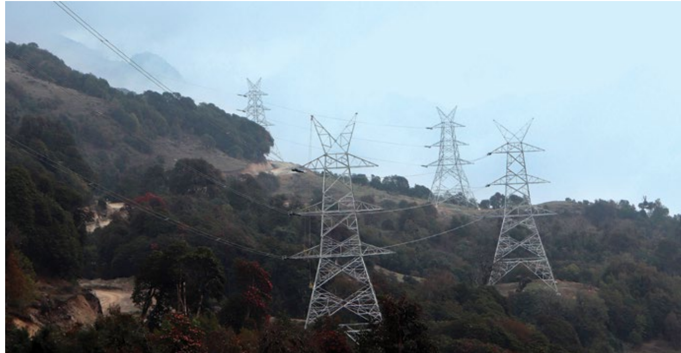
220 kV Basantpur-Dhungesangu Transmission Line, Nepal
