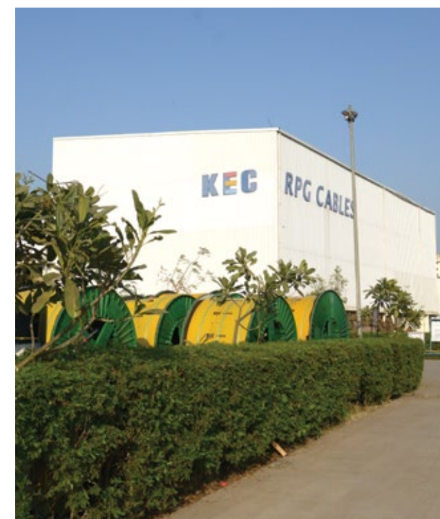
Integrated Cables Manufacturing Plant at Vadodara, Gujarat
