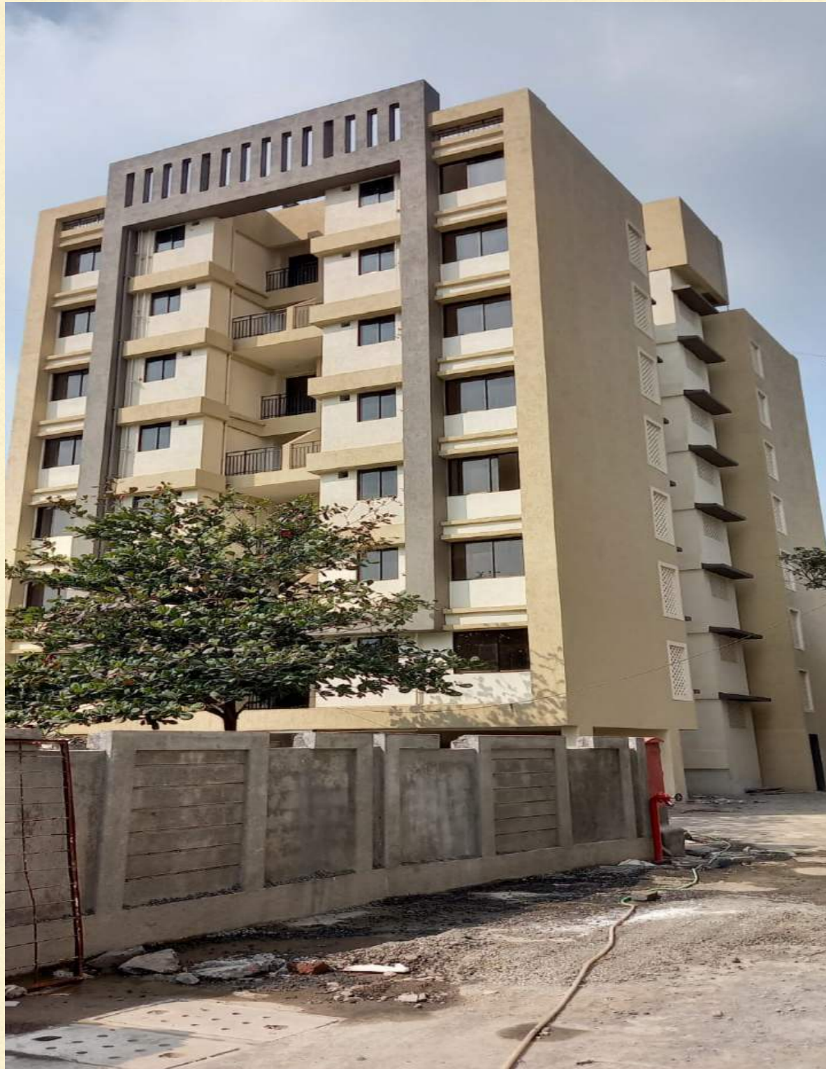
Finishing work nearing completion
