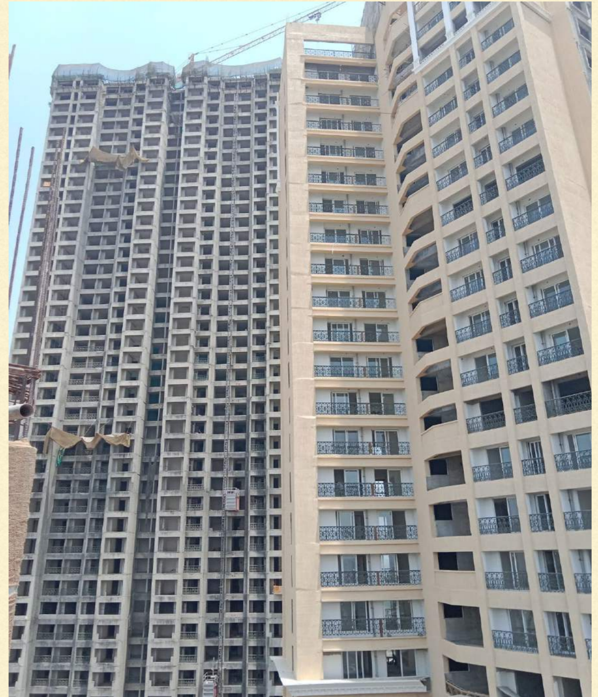
Finishing work in progress beyond 18 th floor in Baraz-I
