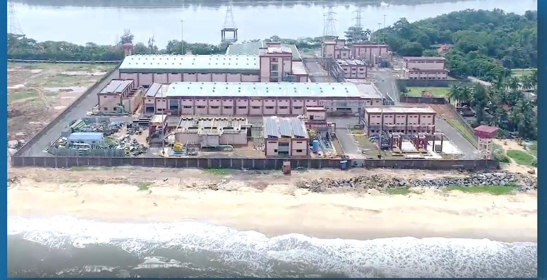
MRPL Desalination Plant, Mangalore, India
