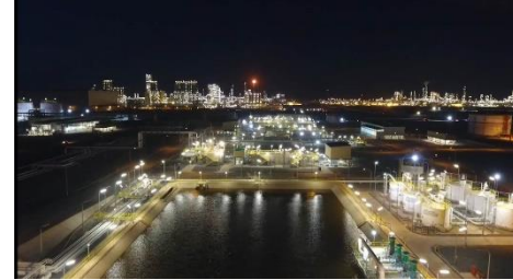
102 MLD Industrial Effluent Treatment Plant for PETRONAS, Malaysia Largest industrial Effluent Treatment Plant in South East Asia
