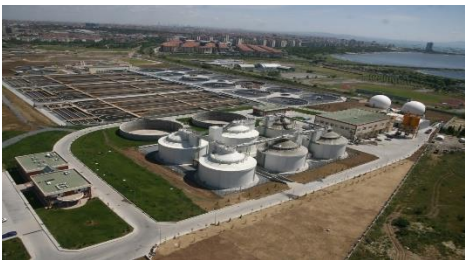
Total City Water Management, Istanbul, Turkey Managed 124 units catering to 16 million population in the Asian and European districts of Istanbul
