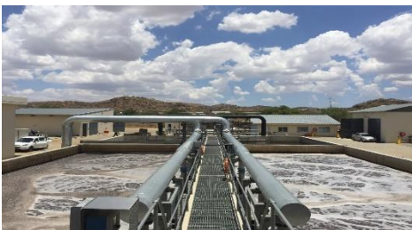
5 MLD Industrial Water Reclamation Plant, Ujams, Windhoek, Namibia First plant of its kind in Namibia, treating effluents from five different production facilities 21 MLD New Goreangab Water Treatment Plant, Windhoek, Namibia First worldwide direct potable water reuse plant.
