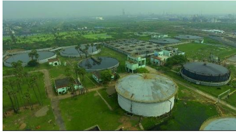
110 MLD Sewage Treatment Plant, Kodungaiyur, Chennai, India One of the most energy efficient and energy neutral STPs in the country
