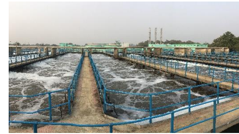
140 MLD Sewage Treatment Plant, Dinapur, Varanasi, India First and largest STP to be inaugurated under 'Clean Ganga' mission
