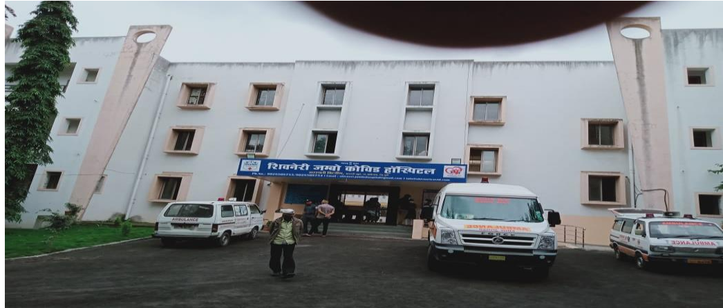
In - conjunction with state government , developed the JUMBO Covid hospital to provide necessary medical support for local residents
