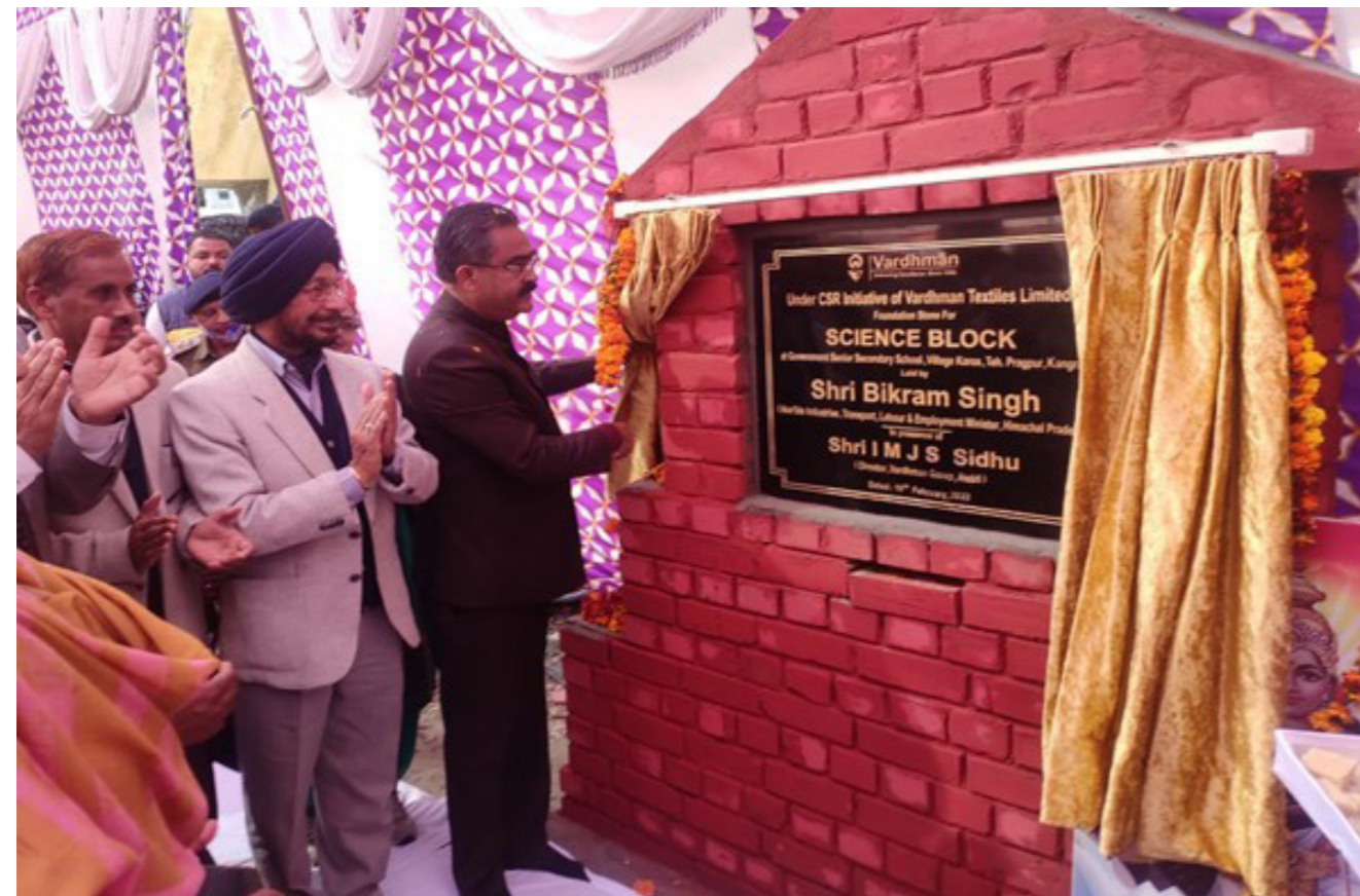
Foundation Stone laid by Industry Minister of HP, Shri Bikram Singh for Science Block at Govt. Sr. Secondary School, Karora, Dist. Kangra
