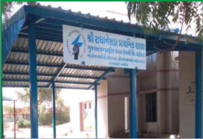
Construction of Shed Shree Raghnesda Primary School
