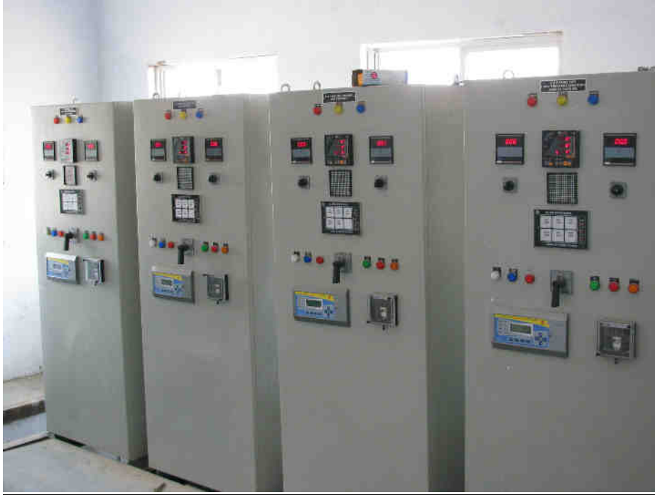
CONTROL & RELAY PANELS
