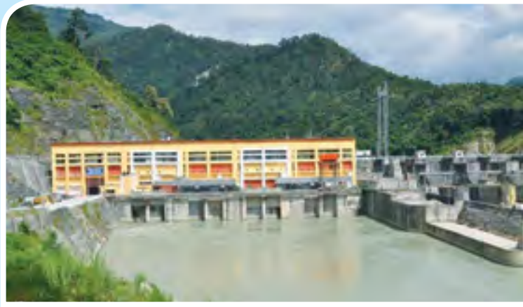
Teesta Low Dam (Stage III) 130 MW Hydro Electric Project in West Bengal Conception to Commission by Texmaco
