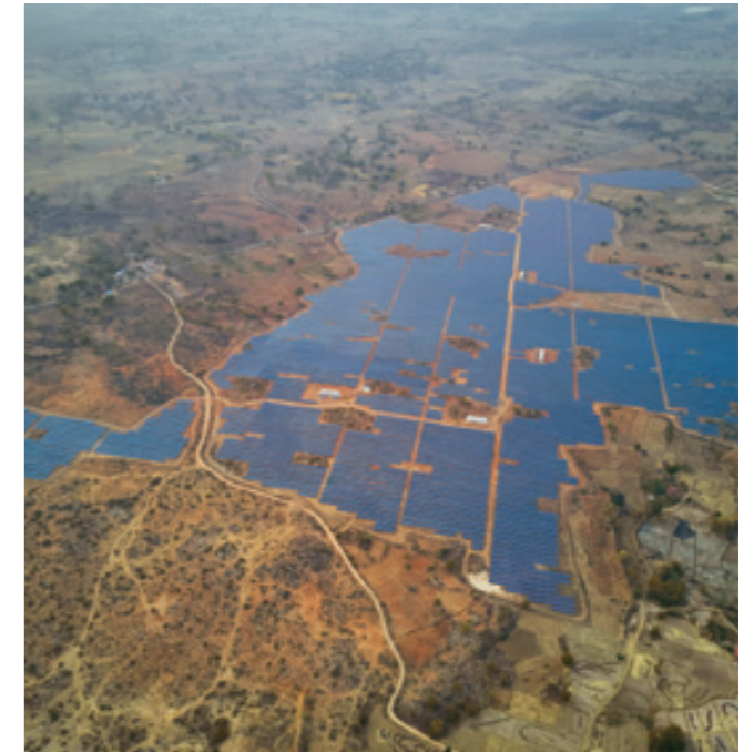
65 MW solar power plant commissioned by Sterling and Wilson Renewable Energy Limited for Energon in Telangana
