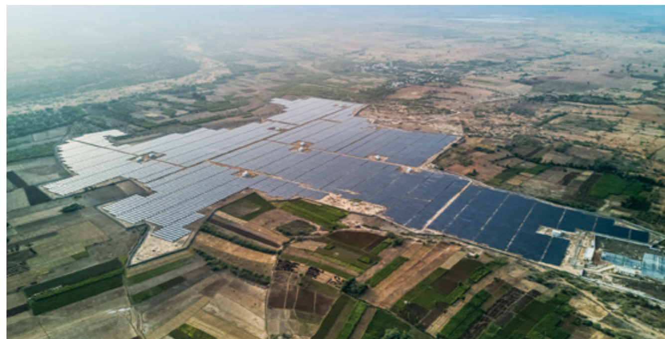
40 MW (AC) Hindupur Solar Park commissioned by Sterling and Wilson Renewable Energy Limited
