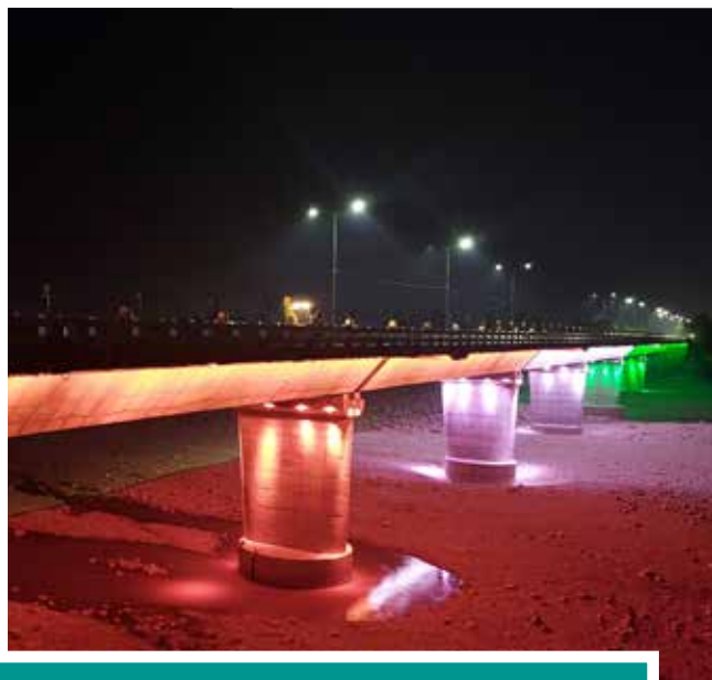
Tawi River Bridge, Jammu
