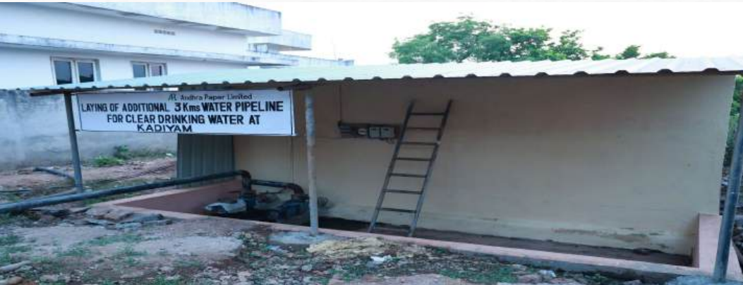
Construction of additional Water Pipelines for clean drinking water at Kadiam
