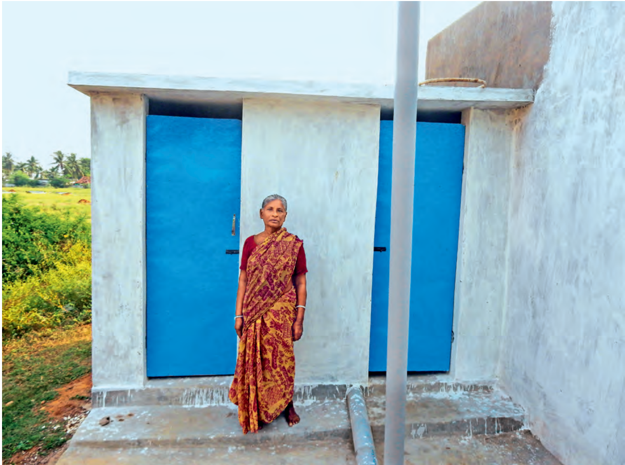
Ms Challapalli Mangathalli in front of her newly constructed toilet
