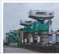
Metro construction works at Kochi, Kerala
