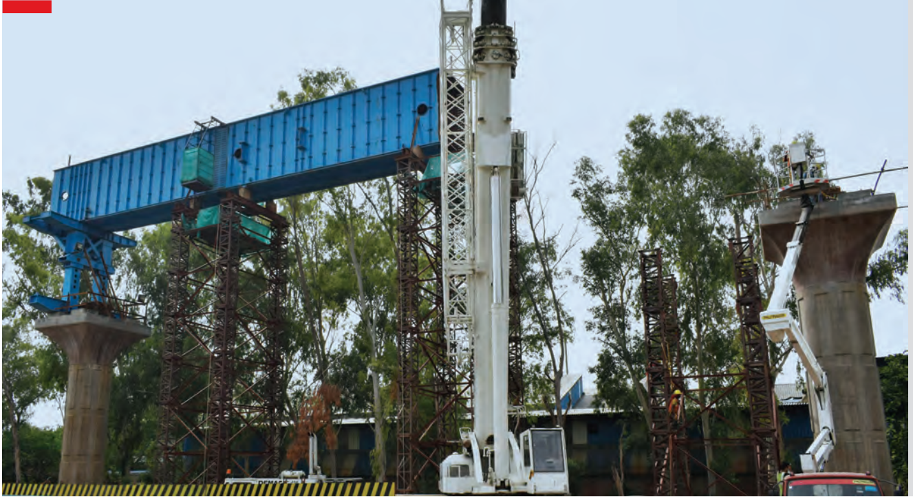
▲ Erection of Launching Girder Box at Delhi-Meerut RRTS project
