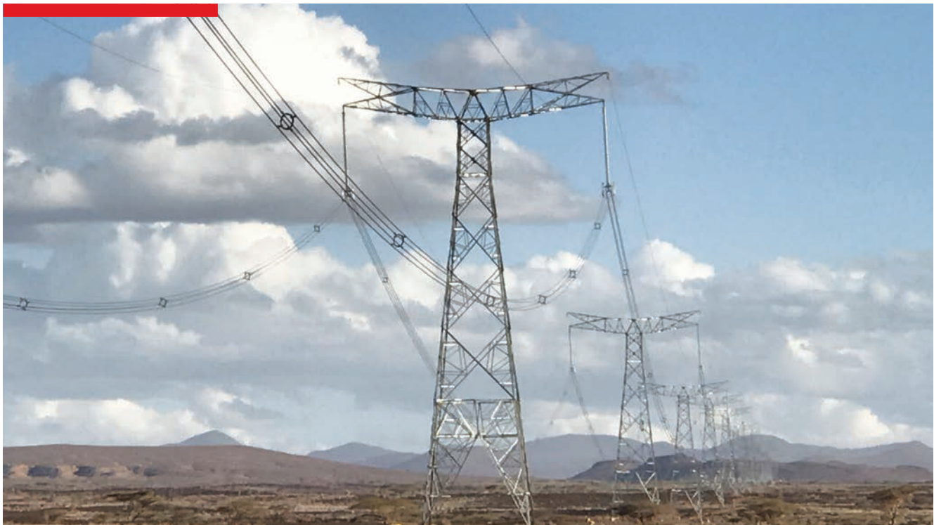
▲ 500 kV HVDC Ethiopia-Kenya Electricity Highway project, first ever 500 kV HVDC transmission line in Africa
