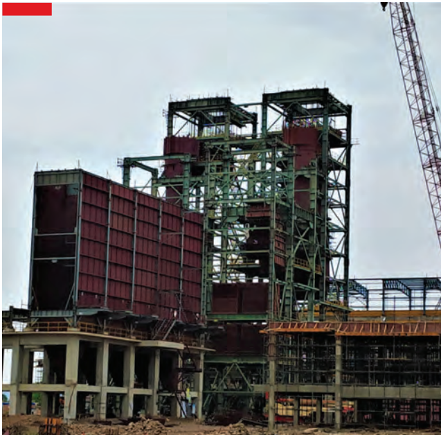
▲ Greenfield cement manufacturing plant at Mukutban, Maharashtra
