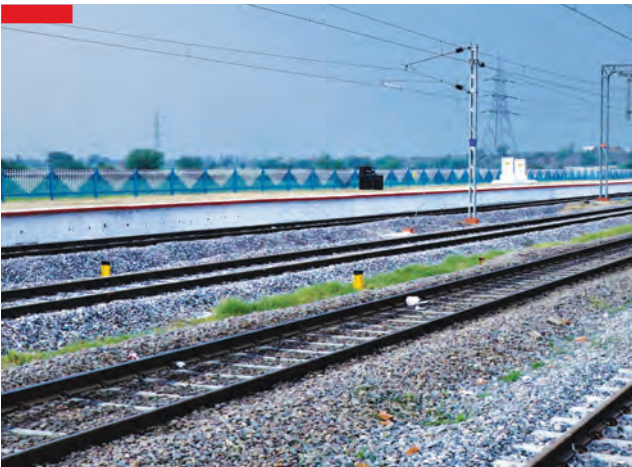
▲ Doubling of tracks between Jhansi-Bhimsen, Uttar Pradesh
