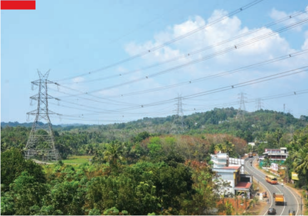
▲ 400 kV Edamon-Kochi Transmission Line for PGCIL, Kerala; First line in the state to be connected to the National Grid
