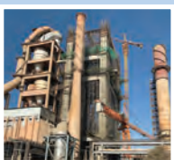
Preheater, cement manufacturing plant at Mundwa, Rajasthan
