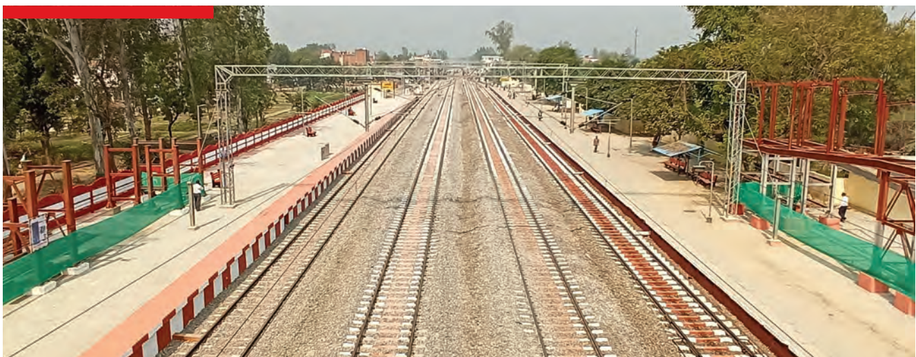
▲ Electrification, track and station works at Amethi, Uttar Pradesh
