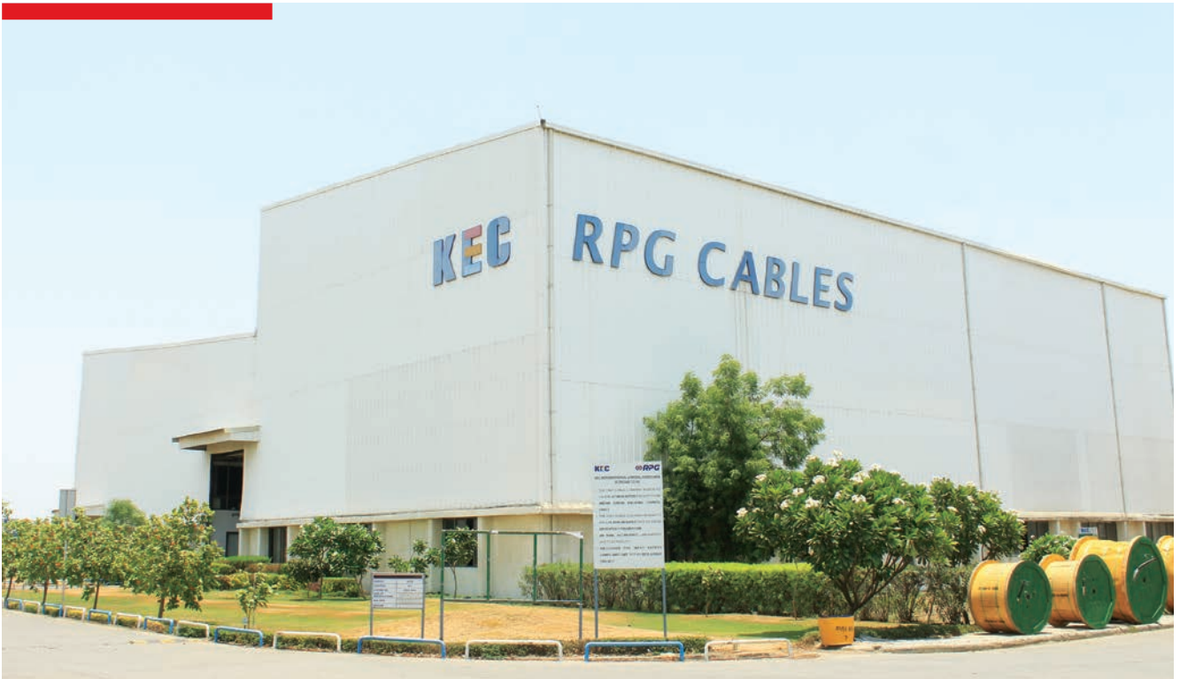
▲ Integrated Cables Manufacturing Plant in Vadodara, Gujarat
