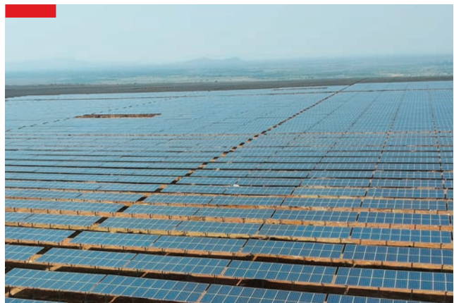
▲ 130 MWp Ground Mount Solar project, Andhra Pradesh
