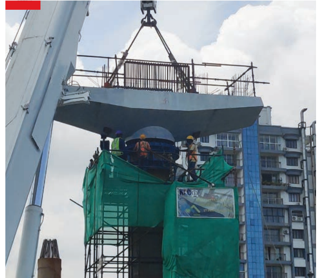
▲ Pier cap erection at Kochi Metro project, Kerala
