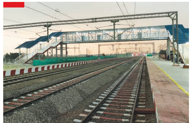
▲ Station works at Gauriganj, Uttar Pradesh
