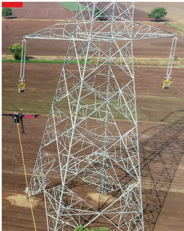
▲ Drone for stringing power conductors
