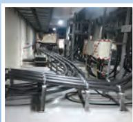
132 kV Underground Cabling works, Oman
