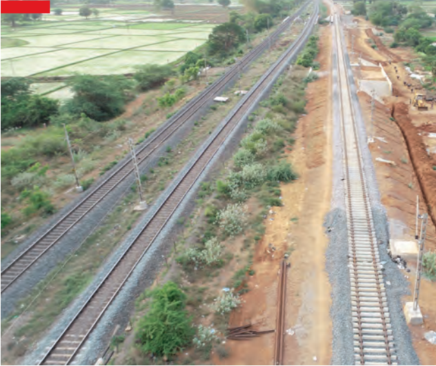
▲ Construction of 3rd line between Gudur-Bitragunta, Andhra Pradesh
