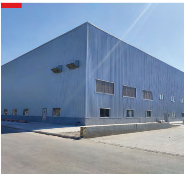
▲ Construction of a factory for an automobile manufacturer at Pune, Maharashtra
