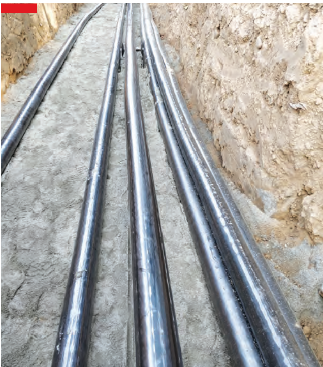
▲ 220 kV Underground Cabling, Chandigarh
