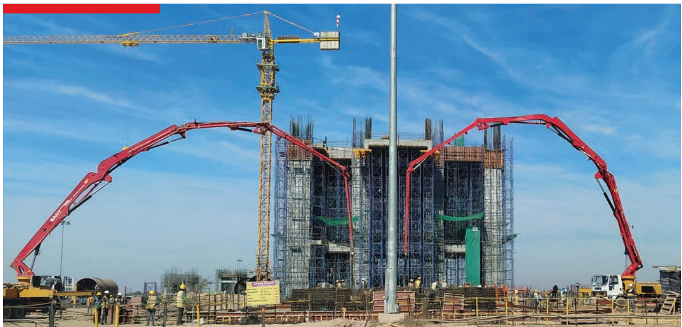
▲ Cement plant for a reputed client in Mundwa, Rajasthan
