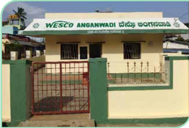
Anganwadi Day Care Centre at Dandeli
