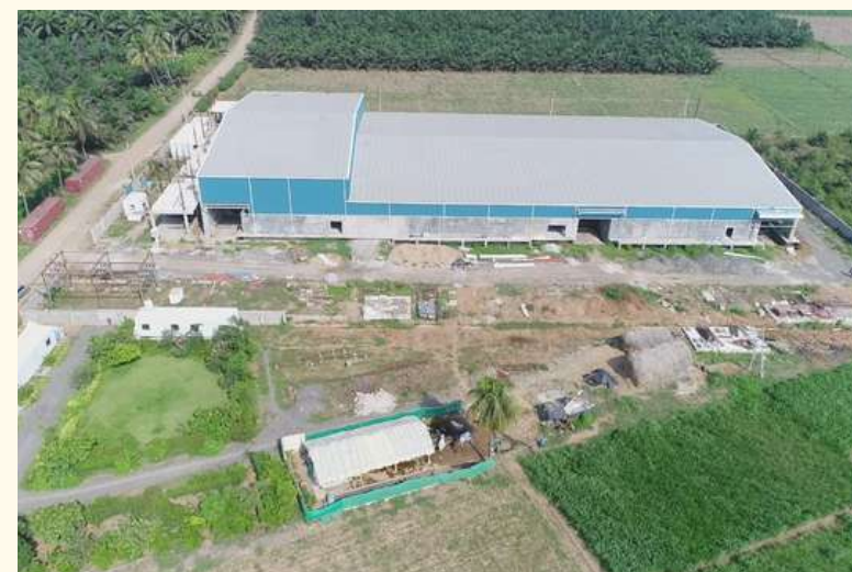
2019 -construction of new facility
