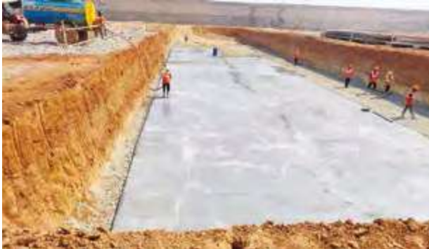
▶ Foundation work is progressing in full swing
