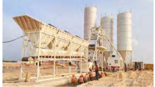
▶ On site construction equipment
