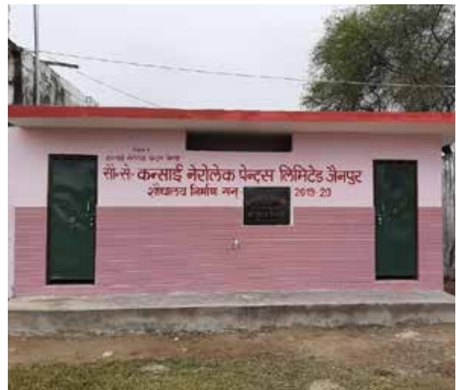
► Construction of toilet in school
