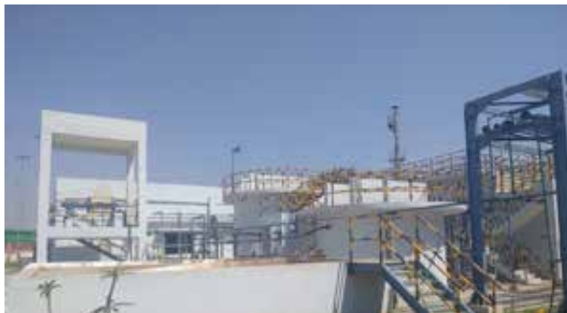
► Zero Liquid Discharge at Goindwal Plant
