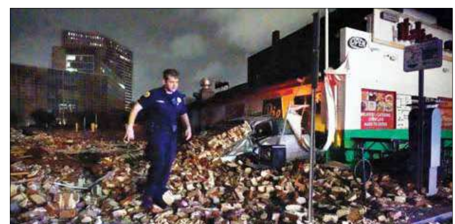
New Orleans Police detective Alexander Reiter, looks over debris from a building that collapsed during Hurricane Ida in New Orleans, Monday
